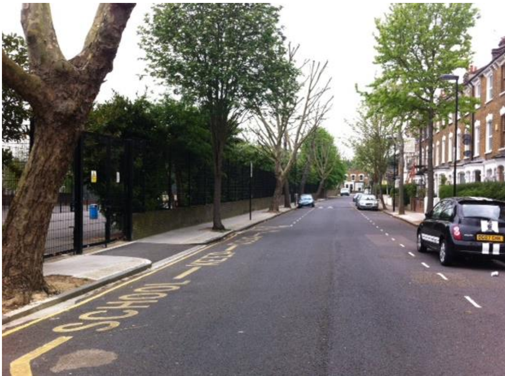
Photo 2: Street view Marriott Road
