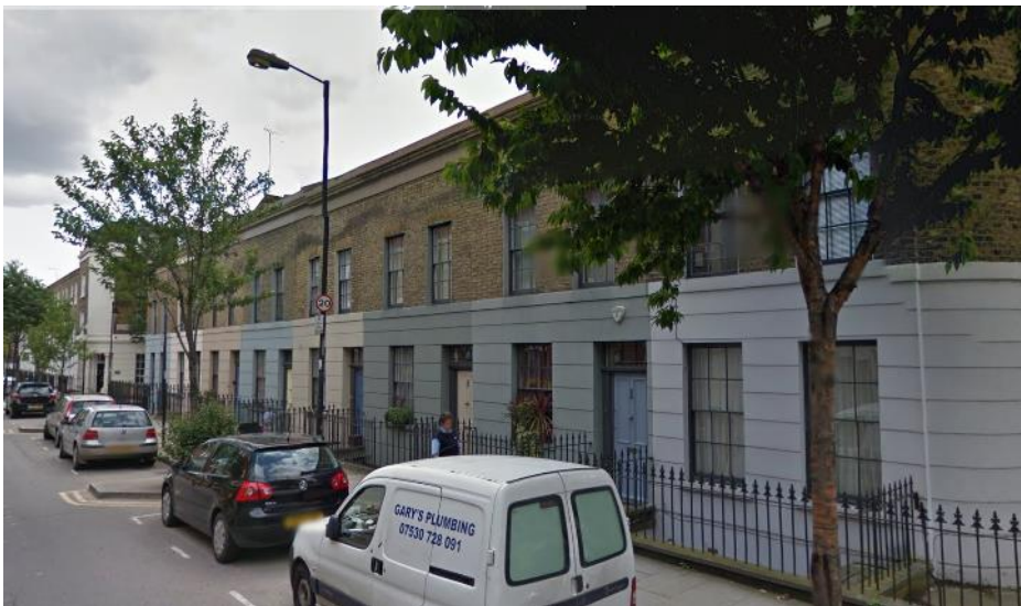
Image 1: Front elevation of the locally listed terrace at Wharfdale Road looking east
