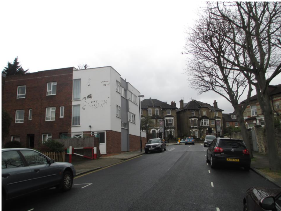
3. View of the rear of the property
