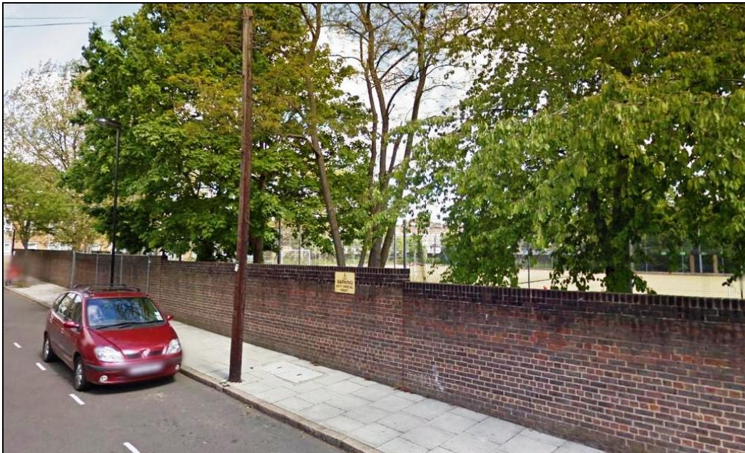
Photo 4: View of existing wall looking north east on Montem Street
