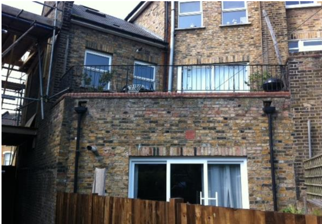
Photo 7: Neighbouring property No. 50d-50f St Thomas Road centre
