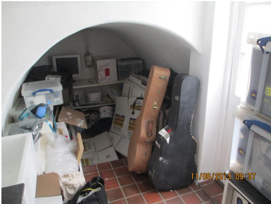
7. The front vault
