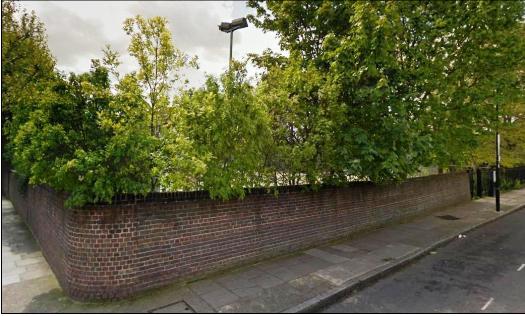
Photo 3: View of existing wall looking north east on Montem Street
