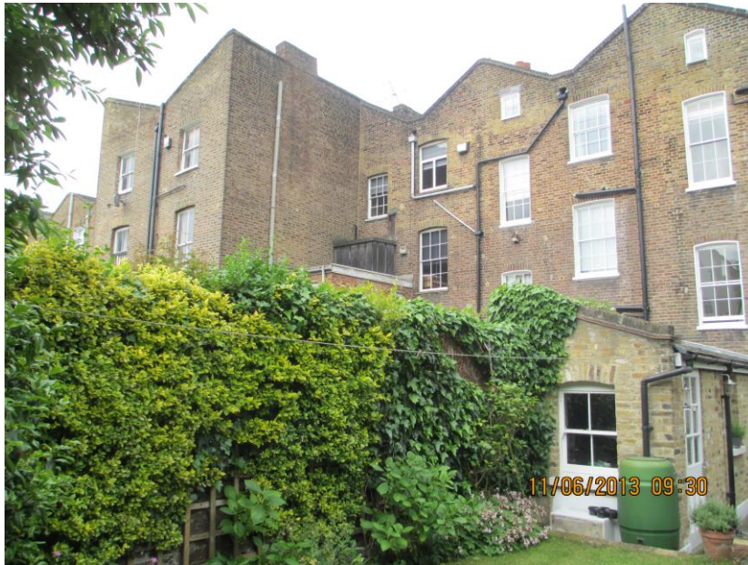
4. Looking towards number 104 Barnsbury Road
