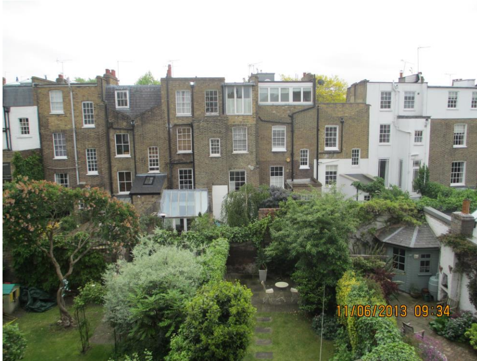
6. The properties to the rear along Cloudesley Road
